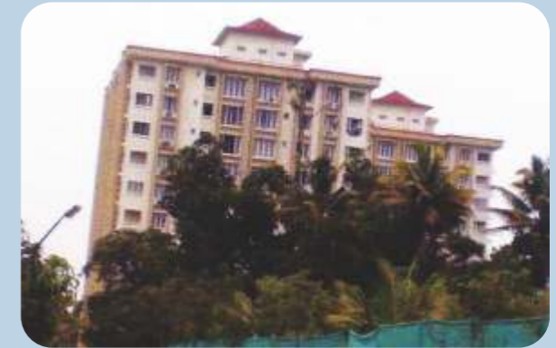
Block 2 at Periyar Heritage Project of M/s. Techni Bharathi Ltd. at Aluva
