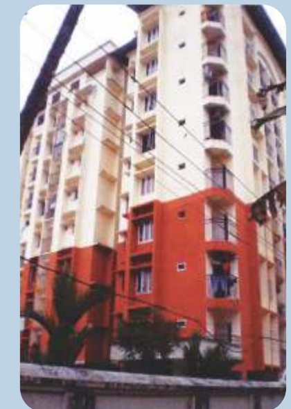
Golden Apple Apartment Project of M/s Apple A Day Properties at Aluva
