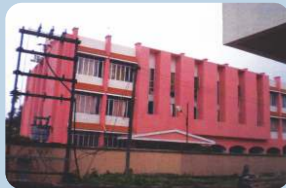
BSNL Administrative Building at Alappuzha
